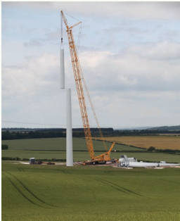
1. The lower sections are connected together
