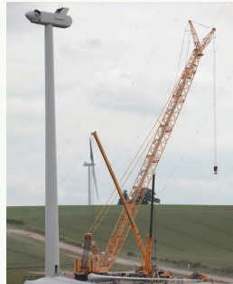
2. The hub and nacelle are put in place.
